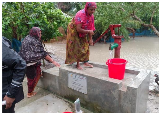
Local caretakers of the deep tubewell using the elevated platform during a flood in Bangladesh. @JakirHossain
