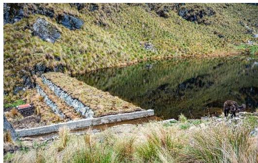
A q'ocha, or small reservoir, that allows rainwater to be stored and infiltrated. @Helvetas
