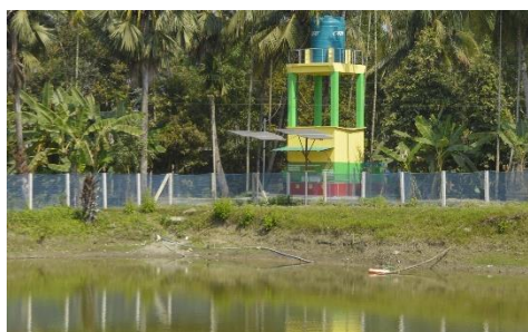
Pond sand filter systems with solar pumps @ShamimHassan
